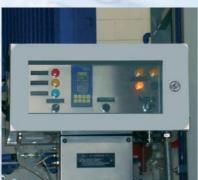
Nitrogen insufflation + Oxygen %02 atmosphere control system.
